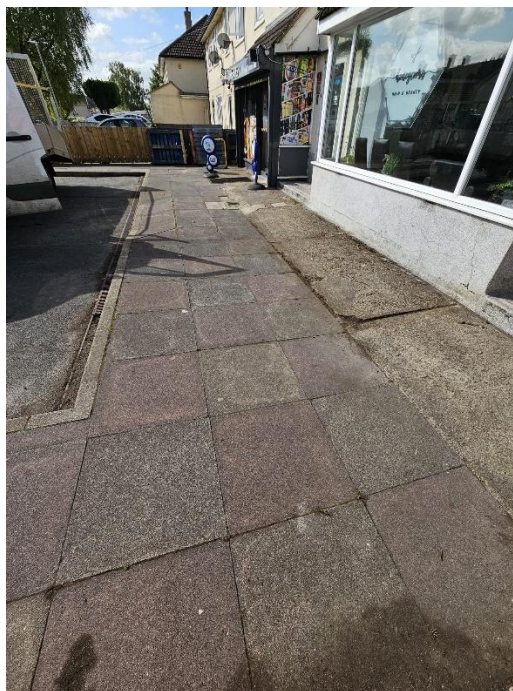
Bourne Road Shops – Tidy up
