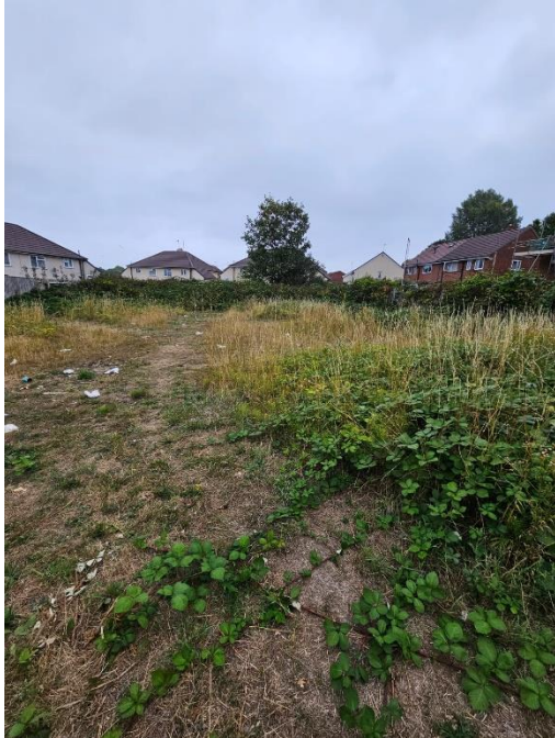
Allington Road Allotment site clearance
