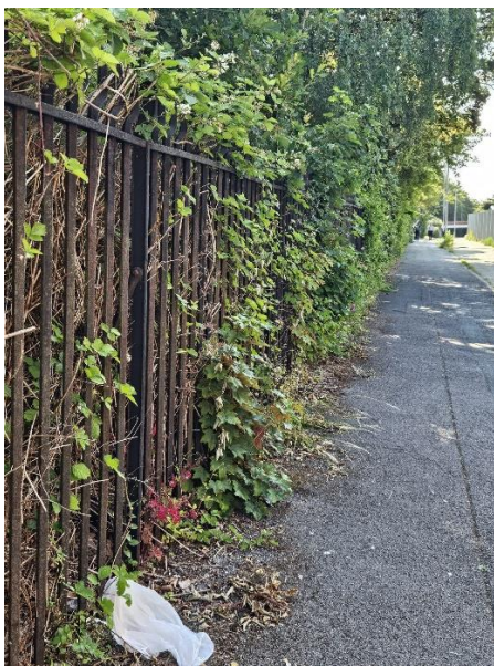
Great Western Flyer – Barge back and weed removal (Before)
