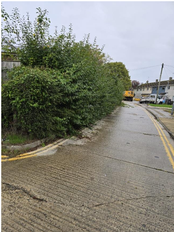
Bremhill Close Hedge encroachment
